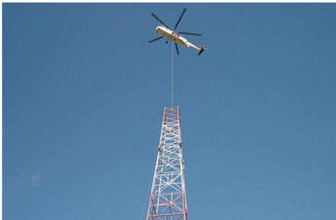
*Rebuilding the WMVP array in Chicago. The 50 kW station on 1000 kHz is owned by ESPN, part of Disney. It had three 500-foot self-supporting towers in a line; Glen Clark & Associates redesigned the array as a 'dog-leg' of guyed towers to help fill nulls. Photos by Glen Clark & Associates*
