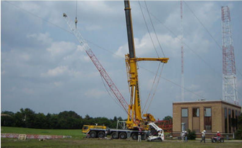
*Rebuilding the WMVP array in Chicago. The 50 kW station on 1000 kHz is owned by ESPN, part of Disney. It had three 500-foot self-supporting towers in a line; Glen Clark & Associates redesigned the array as a 'dog-leg' of guyed towers to help fill nulls. Photos by Glen Clark & Associates*
