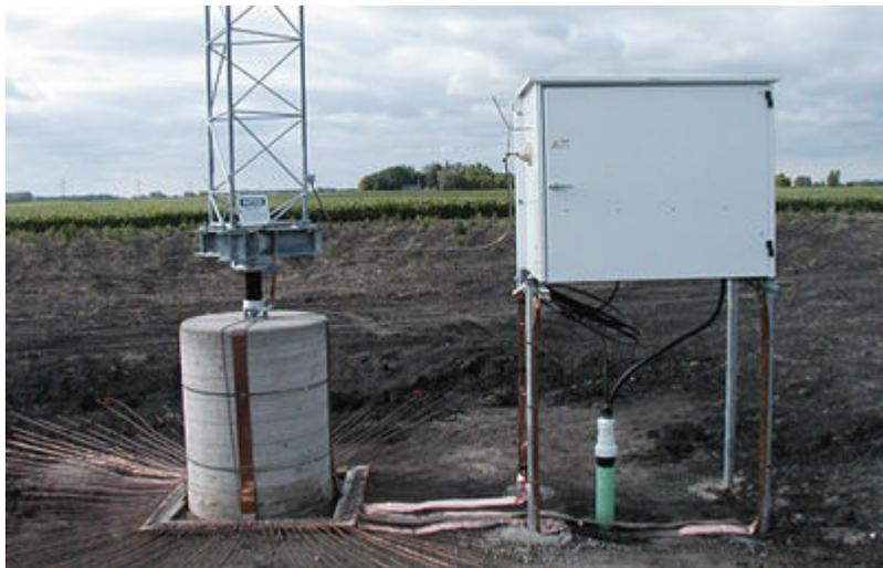
*The challenges facing AM do not mean efforts to improve stations have ceased. Shown are copper radials and ATU cabinet at a new site for KGLB, Glencoe, Minn., west of Minneapolis. Hatfield & Dawson's Tom Gorton tuned up the station on 1310 kHz using 'moment method' computer modeling, as newly allowed under the rules. Photo by Tom Gorton*
